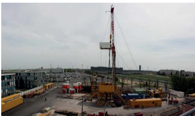
ADP worksite in 2010 (Paris-Orly Airport)
