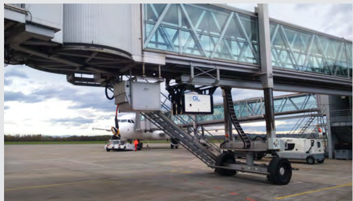
Frequency Converter Passenger bridge mounted.
