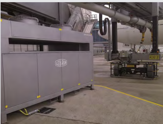
PCA unit at CDG Airport.
