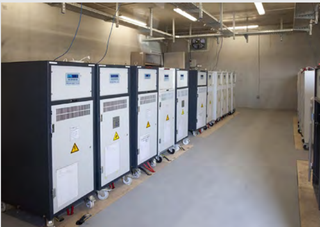
Energy center : Saint Exupéry airport (Lyon).
