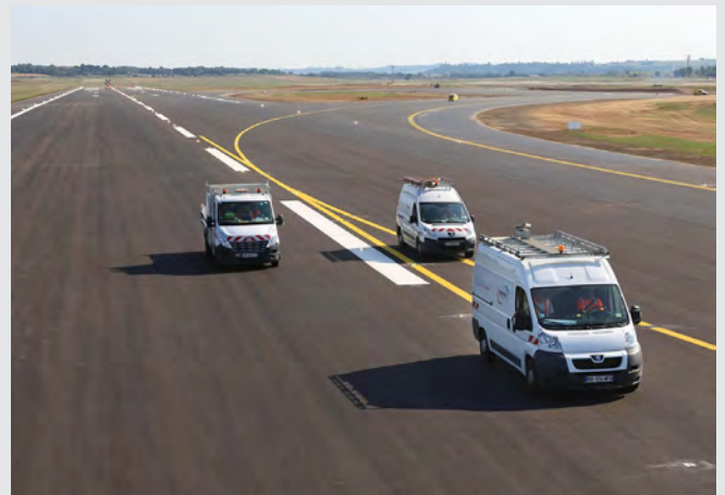
Runway lighting : Saint Exupéry airport (Lyon).
